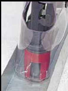
Metal track to concrete
